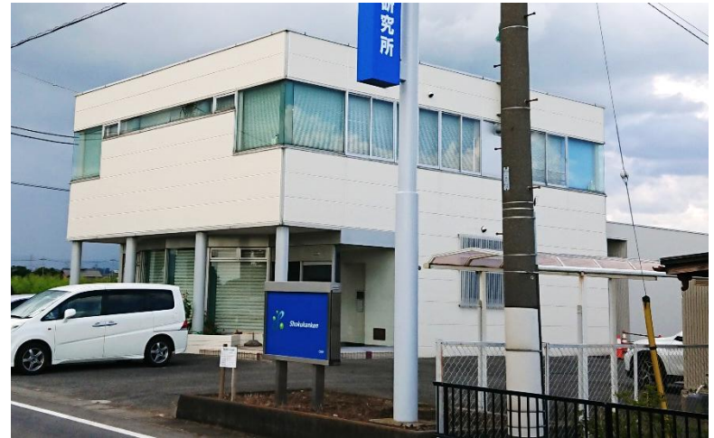
④ Quality control center(GMP)
